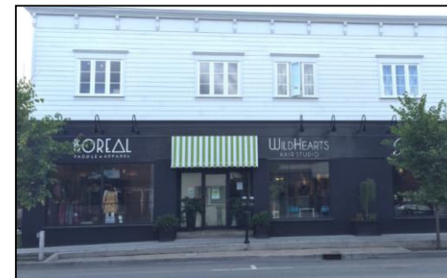
Example of facades before and after improvements in Kenora Image source: City of Kenora, 2017
