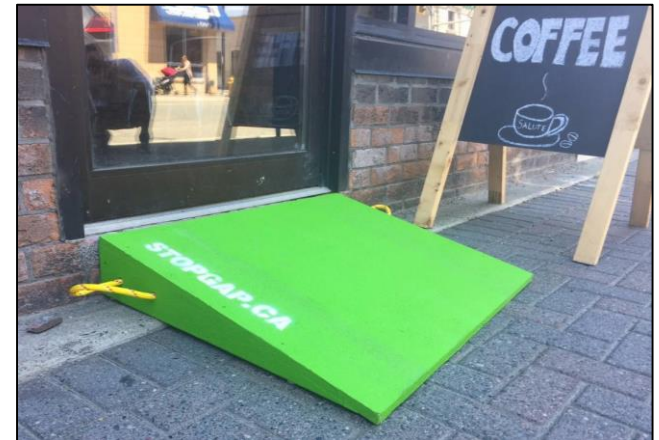
Customized portable ramps as an interim measure to improve accessibility Image source: CBC News, Sudbury, July 5, 2017
